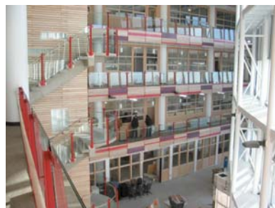
Greenstone Government of Canada Building, Yellowknife
