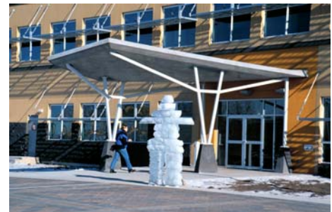
Intuit Canada Headquarters, Edmonton
