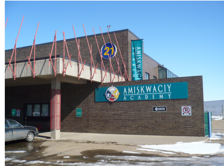
THE SIGN AND THE RED RAILING ARE THE FIRST RECOGNIZABLE FEATURES OF THE SCHOOL BUILDING
